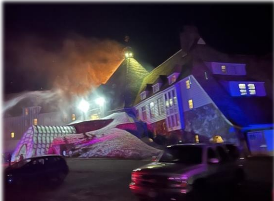
Timberline Lodge Fire
